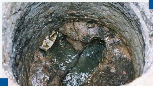
“Brick MH before Poly-Triplex® CIPSL”
