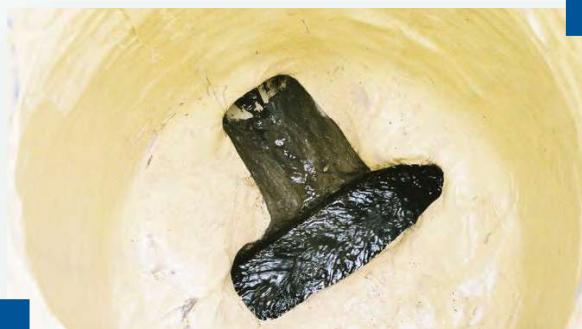
“Brick MH after Poly-Triplex® CIPSL”
