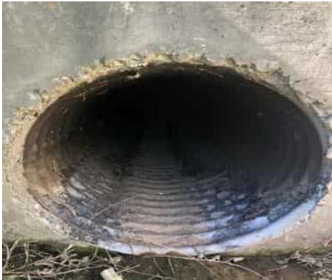
02/23/2021 (NA0017U08 LM:14.306) : LS View: Inside pipe at LS toe.
