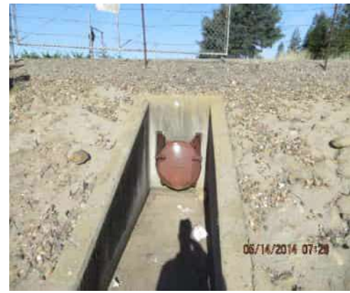
05/14/2014 (NA0017U07 LM:13.819) : Pipe, flap gate, cobble grouted outlet, and concrete headwall on the WS toe.
