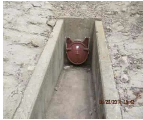
05/20/2014 (NA0017U08 LM:14.324) : headwall and flapgate on WS slope.
