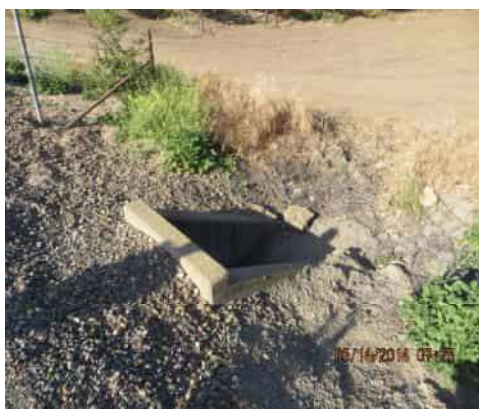
05/14/2014 (NA0017U07 LM:13.819) : Pipe and concrete headwall on LS toe.
