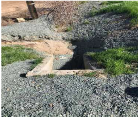
02/23/2021 (NA0017U08 LM:14.324) : LS View: Headwall at LS toe.
