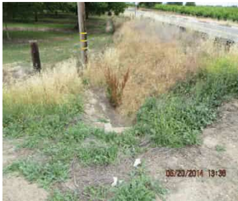
05/20/2014 (NA0017U08 LM:14.324) : Headwall on LS toe.
