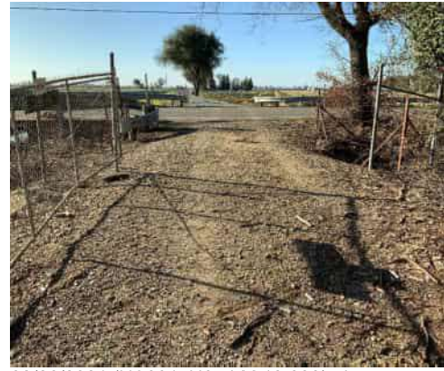
02/26/2021 (NA0017U07 LM:13.838) : Levee crown looking downstream.
