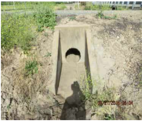
05/21/2014 (NA0017U08 LM:14.306) : Headwall on LS toe.
