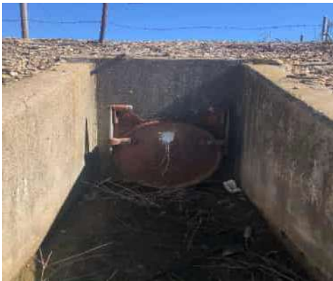
02/23/2021 (NA0017U08 LM:14.306) : WS View: Headwall and flapgate on WS slope.
