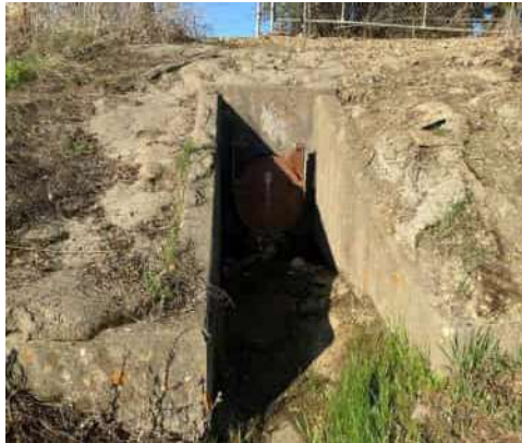
02/26/2021 (NA0017U07 LM:13.838) : WS view: WS headwall and flapgate at toe.
