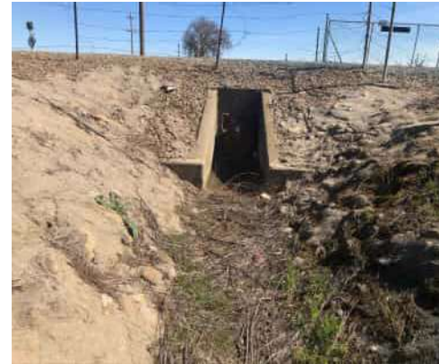
02/23/2021 (NA0017U08 LM:14.306) : WS View: Headwall and flapgate on WS slope.
