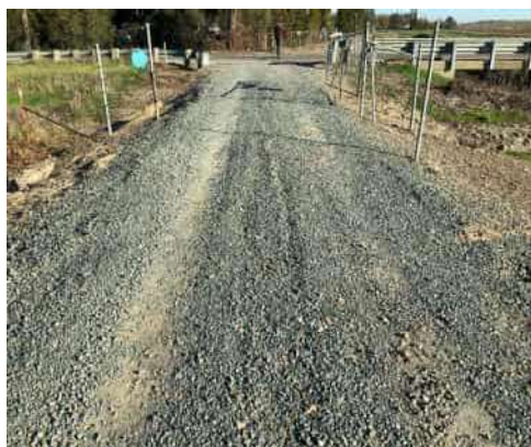
02/26/2021 (NA0017U07 LM:13.819) : Levee crown looking upstream.
