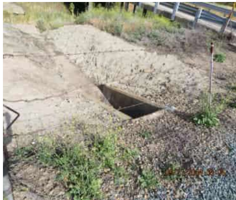
05/21/2014 (NA0017U08 LM:14.306) : Headwall, flap gate, and cobble grouted outlet on the WS slope.
