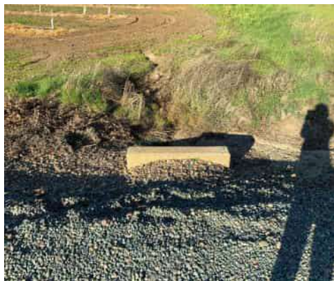
02/26/2021 (NA0017U07 LM:13.819) : LS view: LS headwall at toe from crown.
