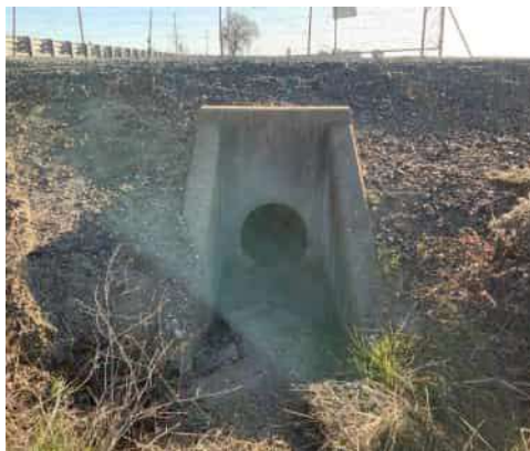
02/26/2021 (NA0017U07 LM:13.819) : LS view: LS headwall at toe.
