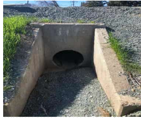
02/23/2021 (NA0017U08 LM:14.324) : LS View: Headwall at LS toe.
