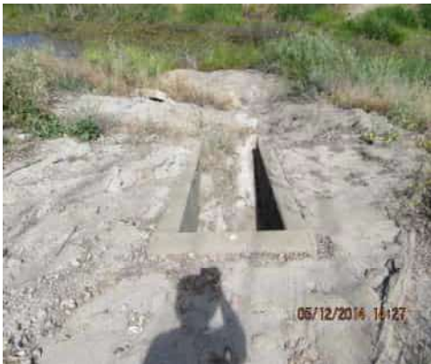
05/12/2014 (NA0017U07 LM:13.838) : Pipe, flapgate, and headwall on WS slope.
