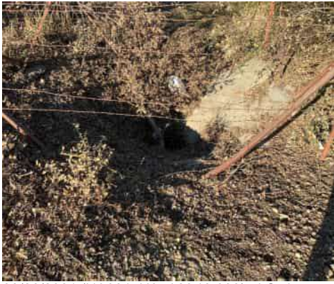
02/26/2021 (NA0017U07 LM:13.838) : LS view: LS toe inlet, surrounded by barbed wire.
