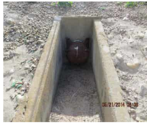
05/21/2014 (NA0017U08 LM:14.306) : Headwall and flapgate on WS slope.
