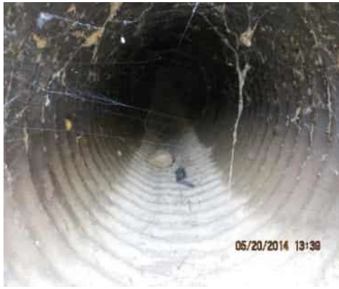
05/20/2014 (NA0017U08 LM:14.324) : Inside pipe at LS toe.
