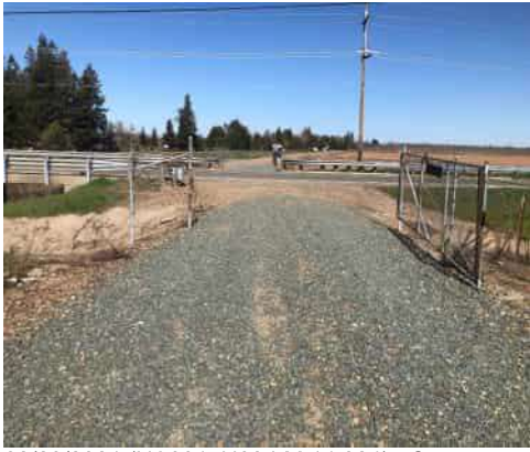
02/23/2021 (NA0017U08 LM:14.324) : Crown Overview - Utility across road.
