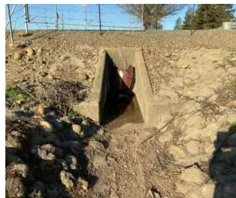
02/26/2021 (NA0017U07 LM:13.819) : WS view: WS headwall and flapgate at toe.
