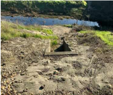
02/26/2021 (NA0017U07 LM:13.838) : WS view: WS headwall at toe from crown.
