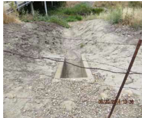
05/20/2014 (NA0017U08 LM:14.324) : Headwall and flapgate on WS toe.
