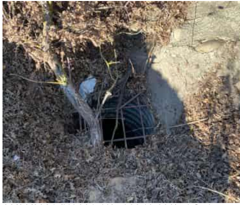
02/26/2021 (NA0017U07 LM:13.838) : LS view: LS toe pipe and inlet.
