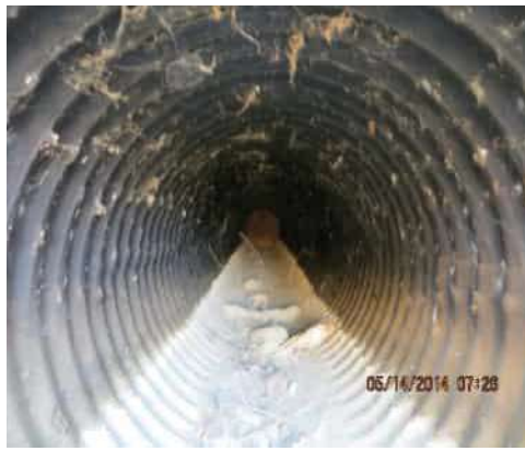
05/14/2014 (NA0017U07 LM:13.819) : Inside pipe from LS toe.
