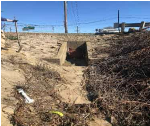
02/23/2021 (NA0017U08 LM:14.324) : WS View: Headwall and flapgate on WS slope.
