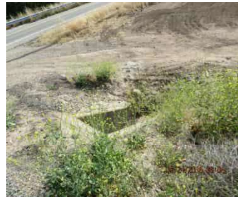
05/21/2014 (NA0017U08 LM:14.306) : Headwall on LS toe.
