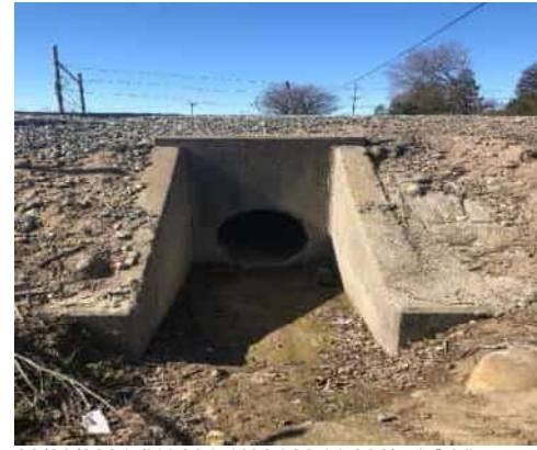
02/23/2021 (NA0017U08 LM:14.306) : LS View: Headwall at LS toe.
