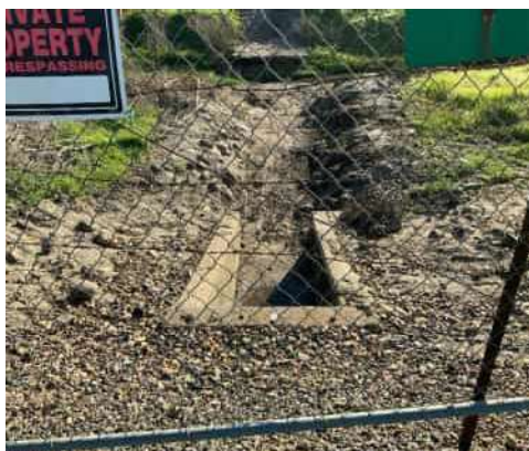
02/26/2021 (NA0017U07 LM:13.819) : WS view: WS headwall at toe from crown.
