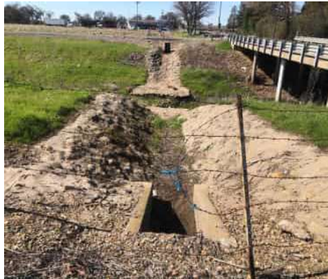
02/23/2021 (NA0017U08 LM:14.306) : WS View: Headwall on WS slope.
