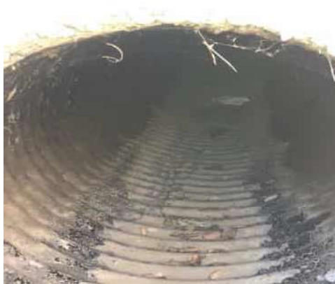
02/23/2021 (NA0017U08 LM:14.324) : LS View: Inside pipe at LS toe.
