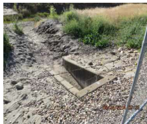
05/14/2014 (NA0017U07 LM:13.819) : Pipe, flap gate, cobble grouted outlet, and concrete headwall on the WS toe.
