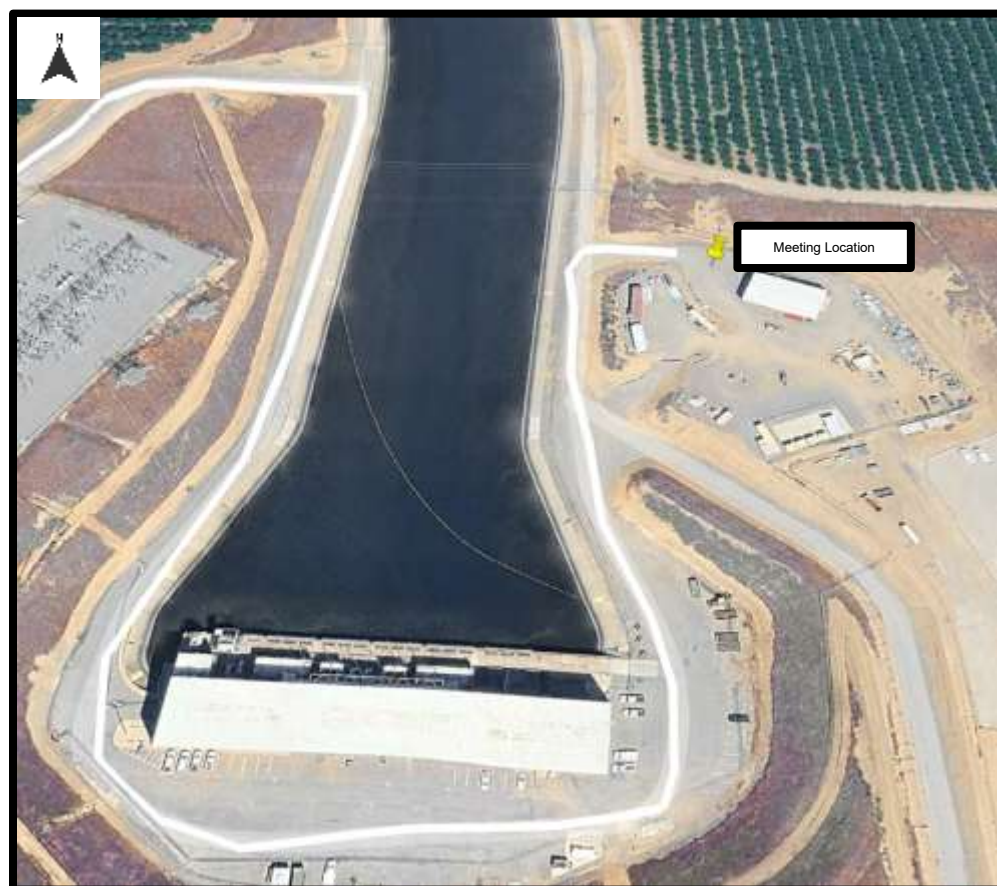
MEETING LOCATION – DOS AMIGOS PUMPING PLANT
