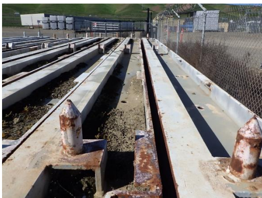
Reference photo of the top of the stop logs.
