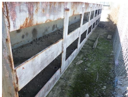
Reference photo of the interior cavities of the stop logs.
