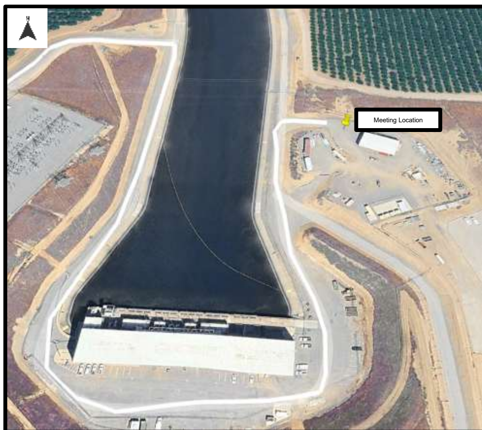
MEETING LOCATION – DOS AMIGOS PUMPING PLANT
