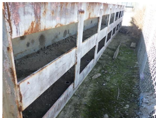
Reference photo of the interior cavities of the stop logs.
