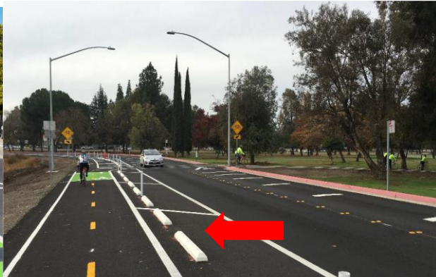
Raised curb and bollard protected
