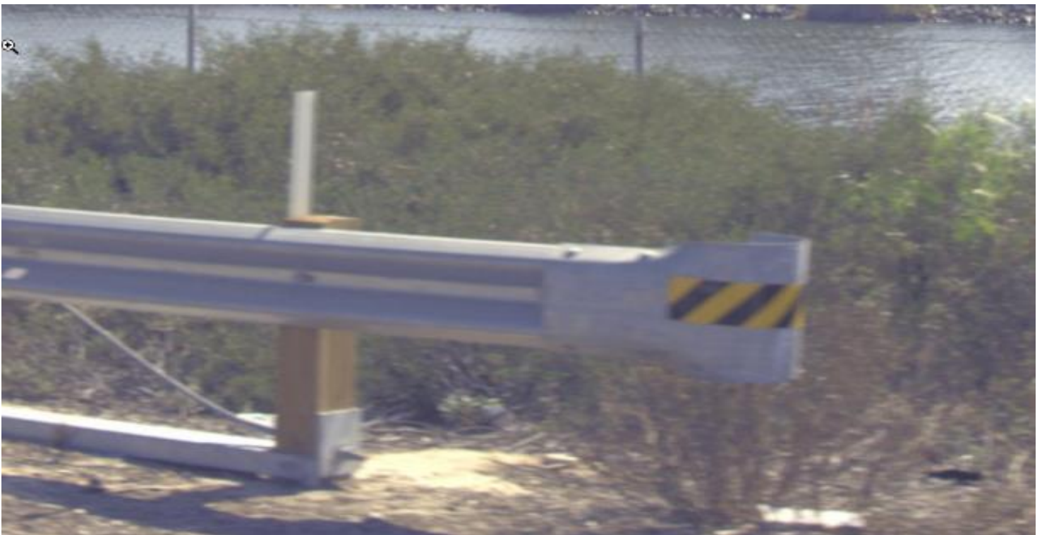
End Anchor Assembly (SFT-M)
