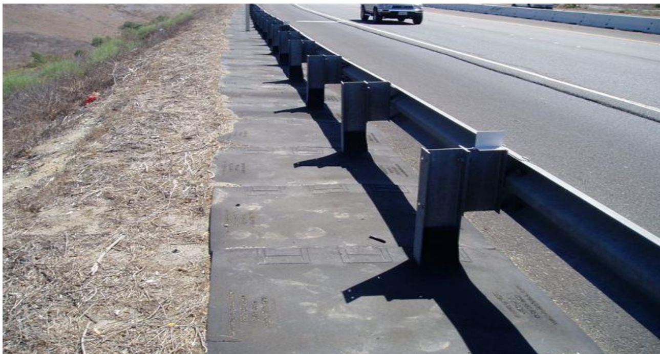
GUARDRAIL MBGR (Metal Beam Guard Railing)
