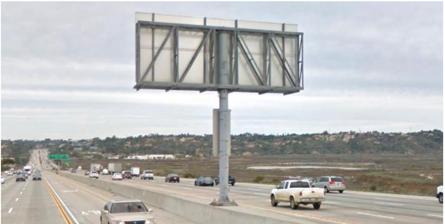
3) ONE POST TRUSS UNBALANCED BUTTERFLY
