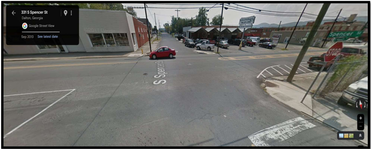
Figure 3 Spencer St Intersection Facing South Before
