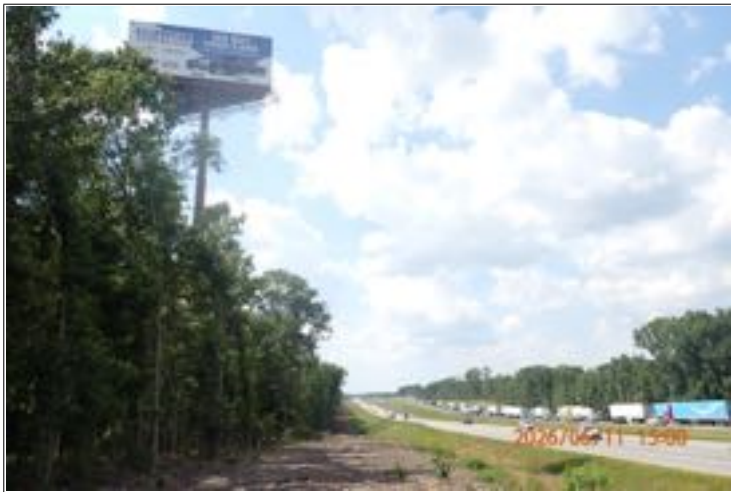
MI1: View of 167'±ht monopole billboard (Permit # D1079) as seen from west side of I-75 along elevated soil area. This is the northernmost billboard on parcel.
