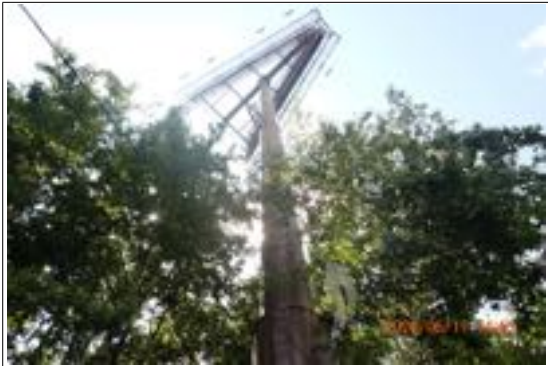
MI2: Photo shows 180'±ht monopole billboard (Permit # D1078) from close proximity.
