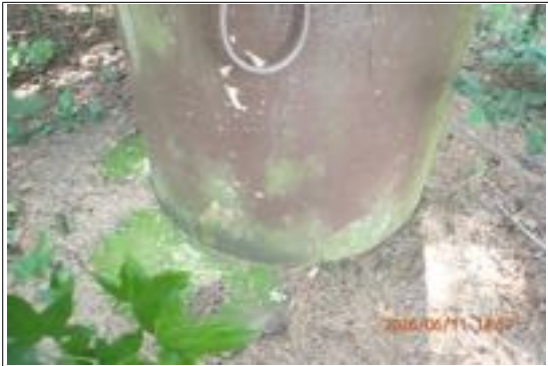
MI1: View of 167'±ht monopole billboard (Permit # D1079) at base.
