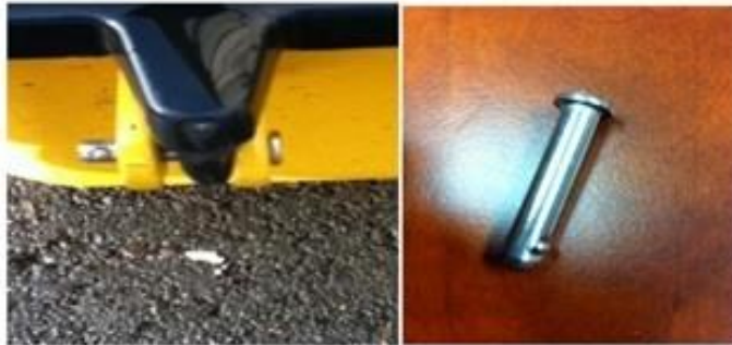
Picture 2 – Door shall have stainless steel hinge pins that are removable without using tools.
