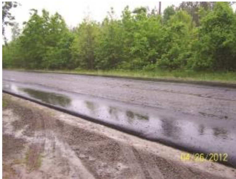
FIGURE E-11 OVERALL SENSORS FACING EAST
