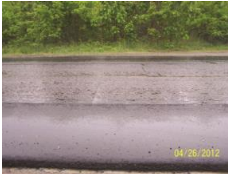
FIGURE E-13 PIEZOS 1 AND 2 LOOKING SOUTH
