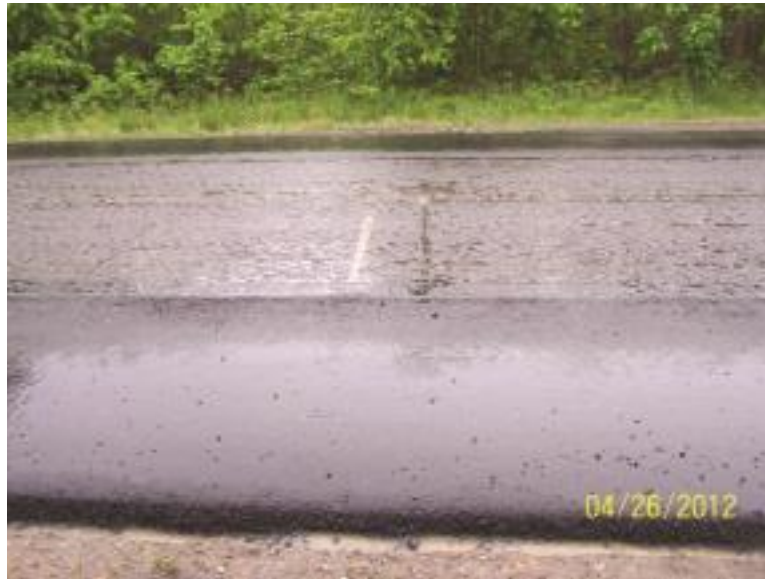
FIGURE E-12 PIEZOS 1 AND 2 LOOKING SOUTH
