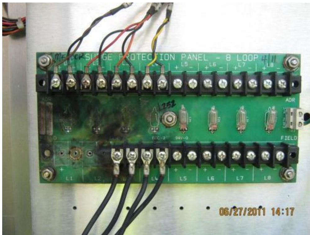
FIGURE F-8 LOOP FIELD CONNECTIONS DESTROYED BY LIGHTNING INDUCED SURGE
