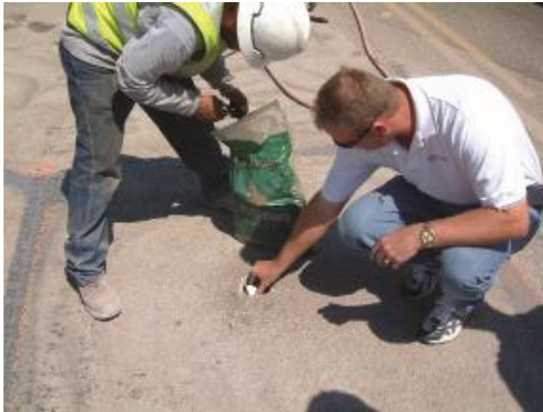
FIGURE 4-7 WIRELESS MAGNETOMETER BEING INSTALLED FOR MOTORIZED TRAFFIC
