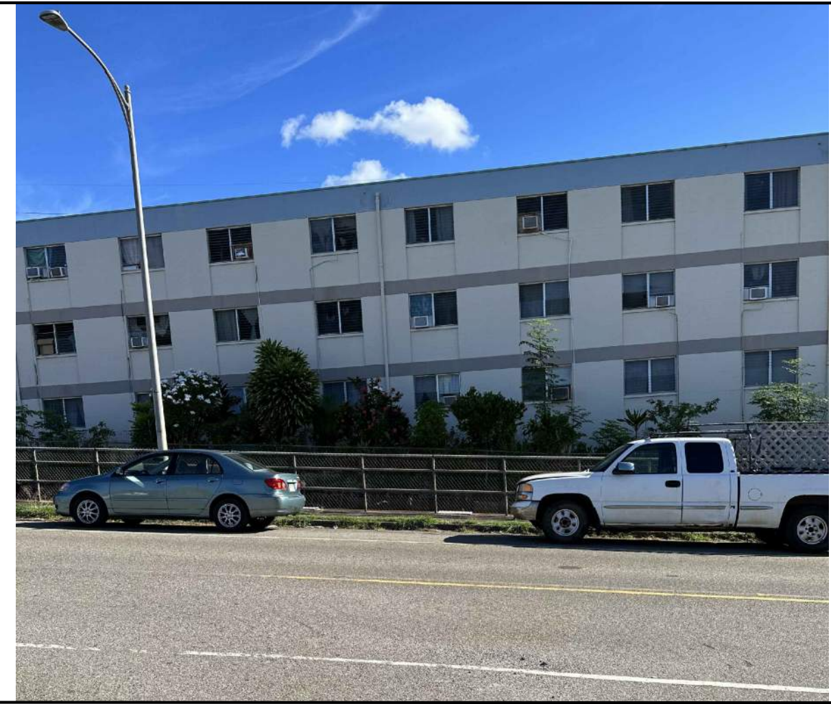
WORK AREA FROM ACROSS KOHOU STREET
