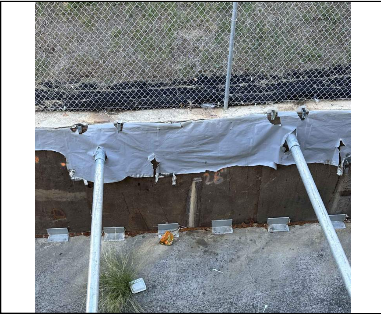
BRACING CONNECTION OPPOSITE ROAD PLATES
