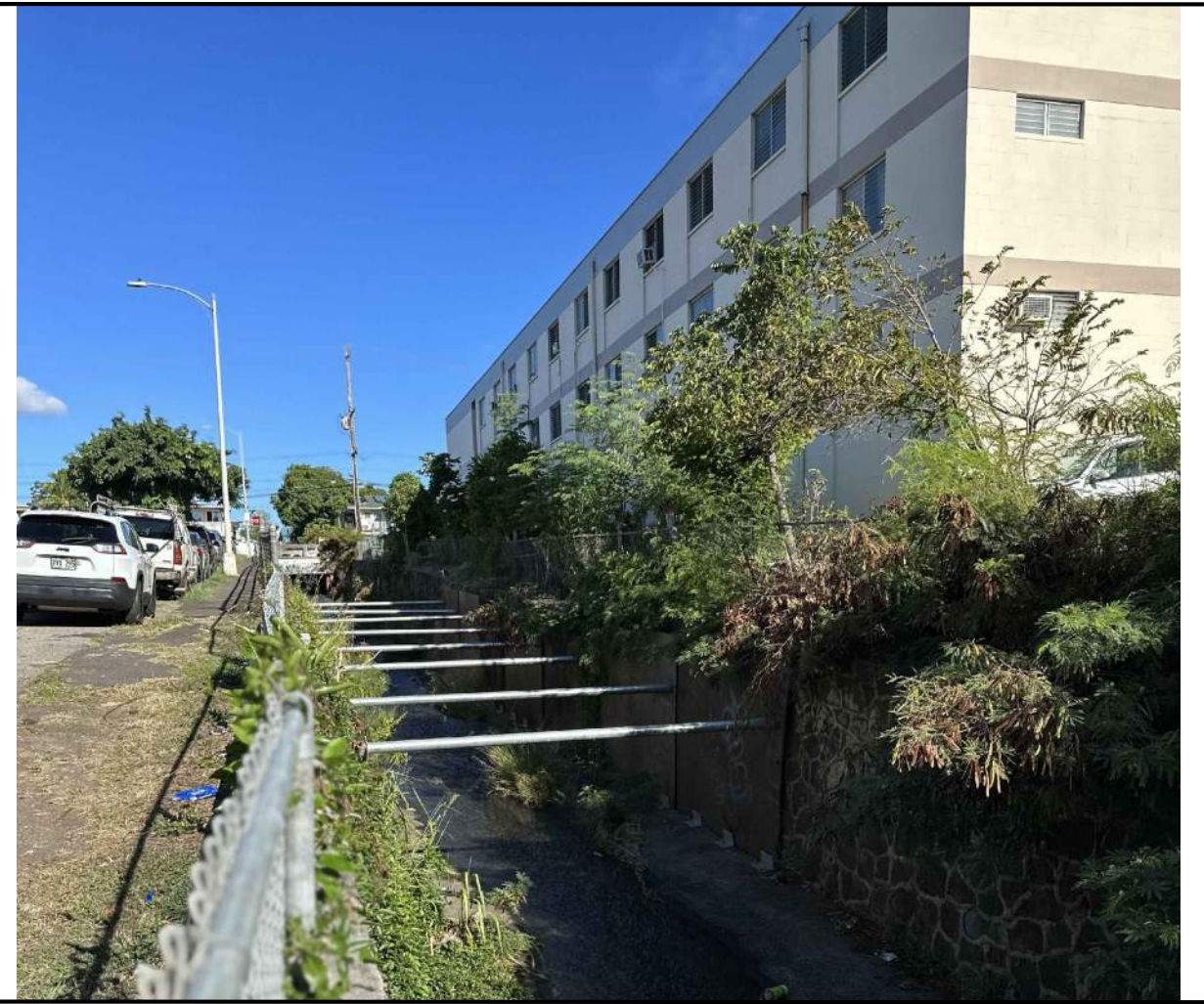
BRACING FROM UPSTREAM
