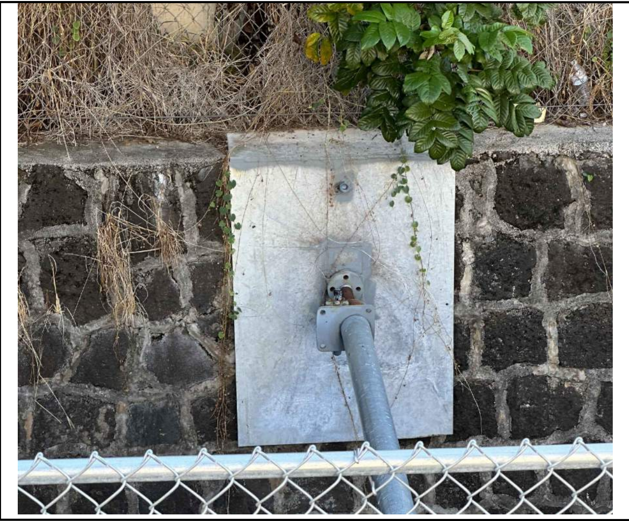
CLOSE UP BRACE CONNECTION
