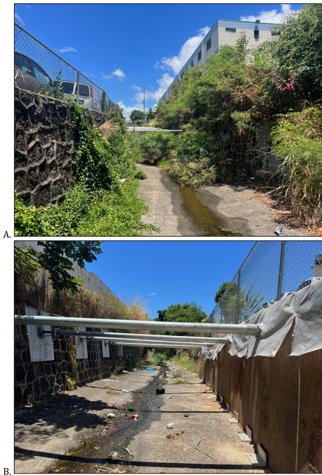
Figure 3. (A) Work area 1 and (B) Work area 2.
