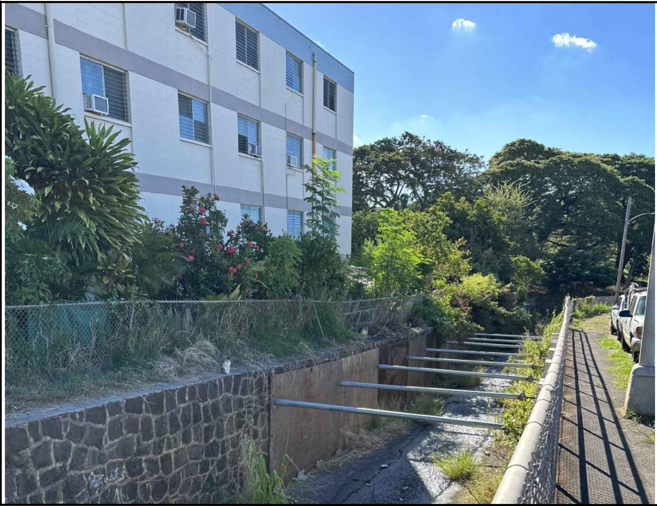
BRACING FROM UPSTREAM
