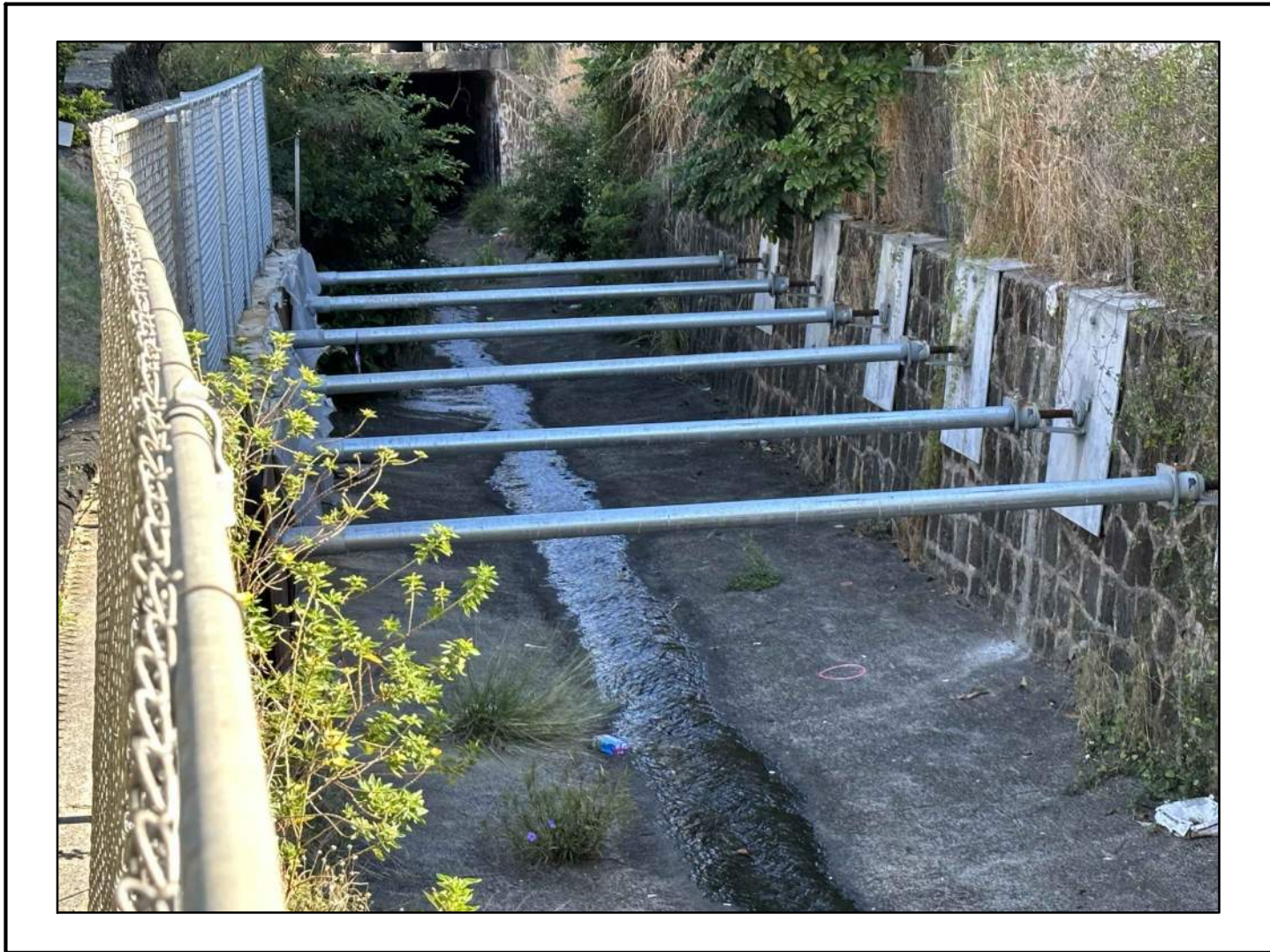
BRACING FROM UPSTREAM
