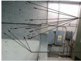
5 DAMAGED BRICK SCALE: NOT TO SCALE REF: A311
