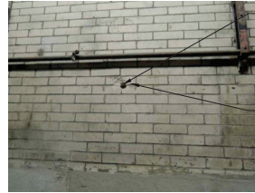
3 ABANDONED PENETRATIONS SCALE: NOT TO SCALE REF: A303
