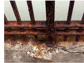
8 DAMAGED CURB SCALE: NOT TO SCALE REF: A303
