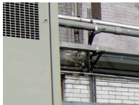
6 DAMAGED CONCRETE SCALE: NOT TO SCALE REF: A203
