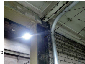
4 ABANDONED PENETRATIONS SCALE: NOT TO SCALE REF: A203
