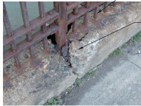
2 DAMAGED CURB SCALE: NOT TO SCALE REF: A203
