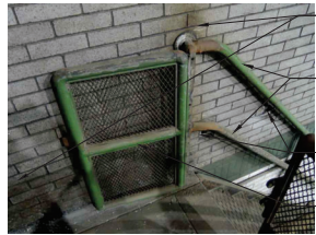
1 LOOSE BRICK SCALE: NOT TO SCALE REF: A213, A214
