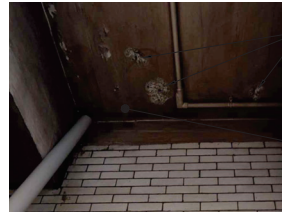
7 SPALLED CONCRETE SCALE: NOT TO SCALE REF: A303
