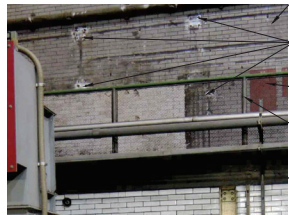
9 ABANDONED PENETRATIONS SCALE: NOT TO SCALE REF: A214
