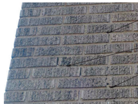
7 CRACKED MORTAR JOINT SCALE: NOT TO SCALE REF: A212
