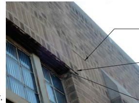
4 A410 DAMAGED LINTEL SCALE: NOT TO SCALE REF: A407
