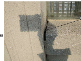
16 A409 OPEN MORTAR JOINT SCALE: NOT TO SCALE REF: A407
