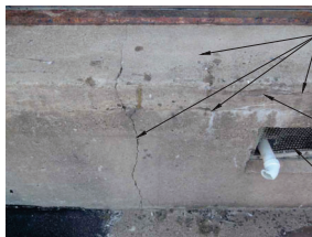
5 A409 CRACKED FOUNDATION SCALE: NOT TO SCALE REF: A407
