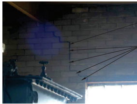
1 A409 CRACKED BRICK SCALE: NOT TO SCALE REF: A403
