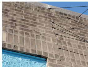
14 A409 CRACKED BRICK SCALE: NOT TO SCALE REF: A407
