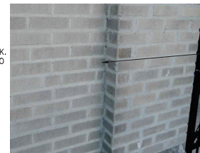
8 A409 CRACKED MORTAR JOINT SCALE: NOT TO SCALE REF: A407
