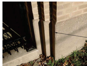
15 A409 CRACKED FOUNDATION SCALE: NOT TO SCALE REF: A407
