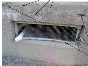
6 A409 CRACKED FOUNDATION SCALE: NOT TO SCALE REF: A407
