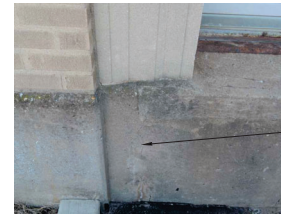
4 A409 CRACKED FOUNDATION SCALE: NOT TO SCALE REF: A407
