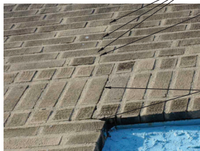
13 A409 CRACKED MORTAR JOINT SCALE: NOT TO SCALE REF: A407
